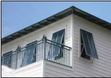
**Figure 4-10. Bahama shutters made from durable extruded aluminum components add “Island” flair to a home and provide opening protection.**
